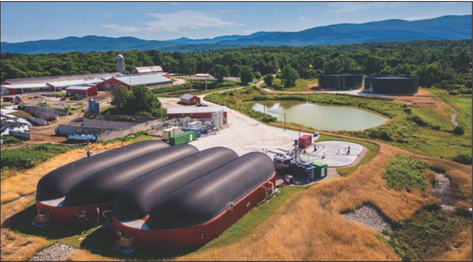
VANGUARD RENEWABLES' FARM Powered anaerobic digester at the Goodrich Family Farm in Salisbury processes manure from dairy cows and other sources into biogas that can be used to make electricity.
