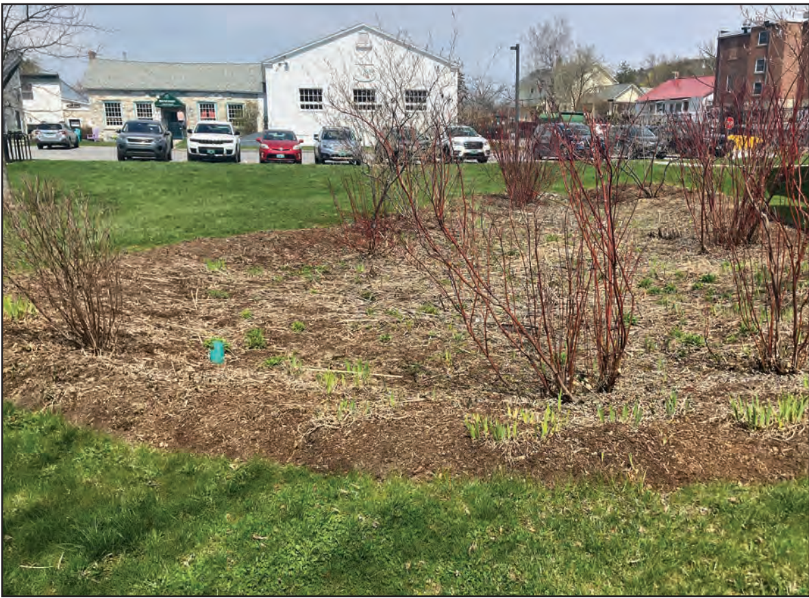
THIS RAIN GARDEN in Middlebury’s Marble Works complex is classically situated in a low-lying spot where it can collect and absorb rainwater and also filter some contaminants out of the water that runs off the nearby parking lot.
