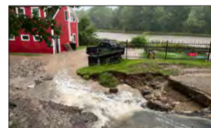
A LARGE SECTION OF Route 116 in Middlebury collapsed early Friday morning after water from a heavy rainstorm that had been pouring for days. The road, which was still pouring a year after the rainstorm of Friday afternoon, was closed by the weather, and temporary signs were set to direct water over the closed roadway and to direct driving water around the water.
