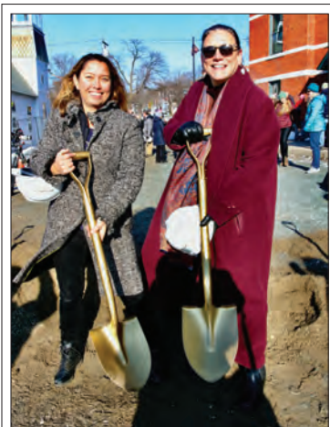
Digging into the future TOWN HALL THEATER Executive Director Lisa Mitchell and Middlebury College President Laurie Patton mark the symbolic start to the next phase of the Middlebury arts institution's growth, as they take part in a THT addition groundbreaking on Tuesday. See more photos on Page 11A. Independent photo/Steve James
