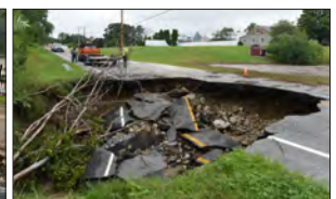
A LARGE SECTION OF Route 116 in Middlebury collapsed early Friday morning after water from a heavy rainstorm that had been pouring for days. The road, which was still pouring a year after the rainstorm of Friday afternoon, was closed by the weather, and temporary signs were set to direct water over the closed roadway and to direct driving water around the water.
